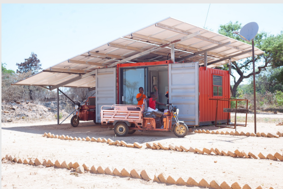
Figure 3-2 Integrated PV-charging-battery storage & swap station
